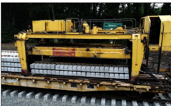
The photos above showcase the TCM installing new track in Berlin
