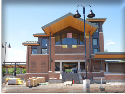
Construction at Berlin Station
