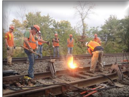
Welding along the track in North Haven
