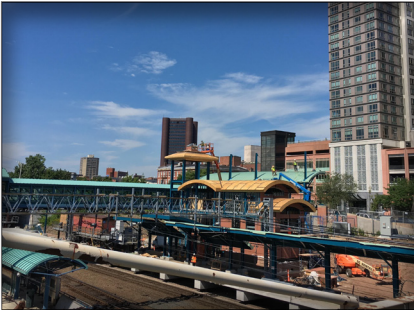
Construction at State Street Station in New Haven
