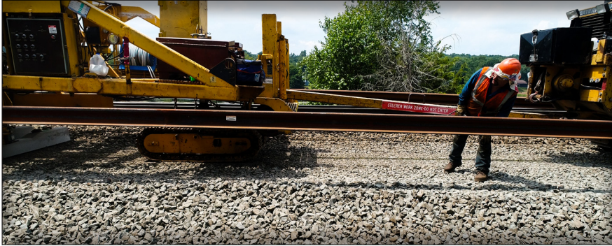
Track Construction Machine laying new track in Berlin
